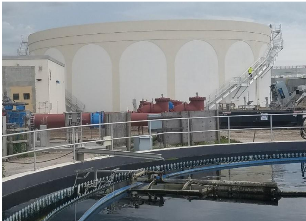
Figure 3-4. Largo equalization tank constructed to reduce peak flow conditions associated with wet weather events.
