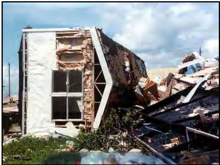
Storm damage to mobile home
