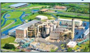
Garbage in Pinellas County is taken to the Solid Waste Disposal Complex, where 80 to 90 percent of it is burned as fuel in the County's Waste-to-Energy (WTE) facility. Pinellas County's WTE facility produces enough electricity to power 45,000 homes each day. The gas produced is cleaned by state-of-the-art pollution control systems.
