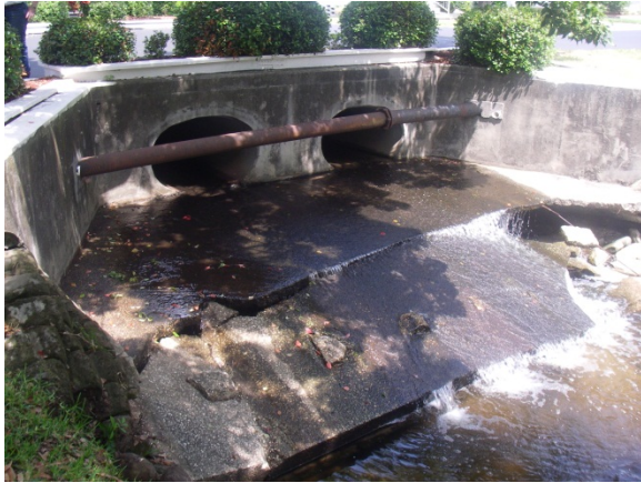
Oak Crest culverts at Twin Oaks Drive (downstream)
