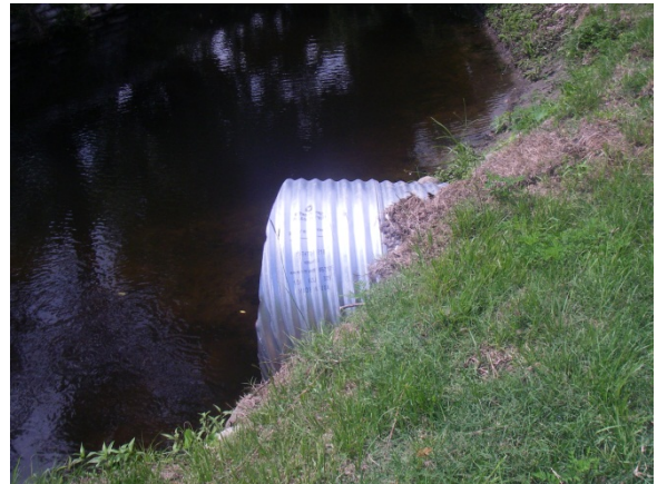
Barrington Trace Berm (Future Roadway) Culvert
