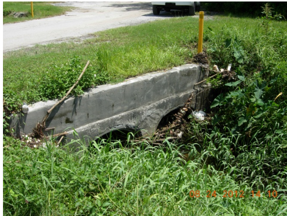
City of Largo Maintenance Facility Culverts
