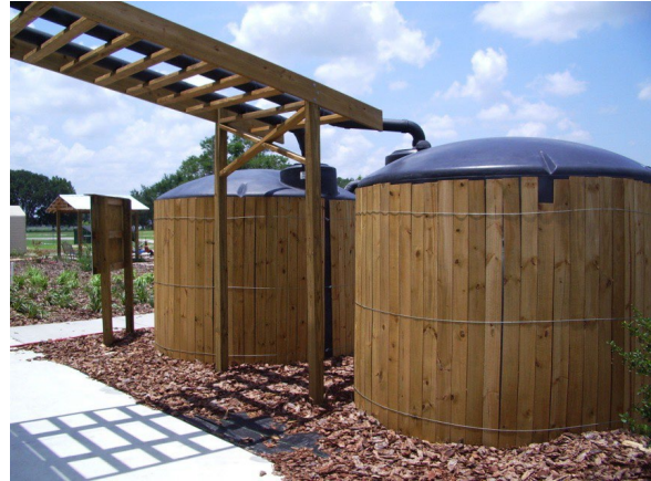
A rainwater harvesting cistern used for irrigation.
