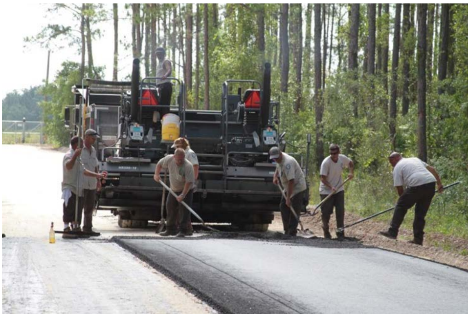
Photo 2-6 Hot mix asphalt pavement incorporating processed WTE bottom ash as a partial aggregate replacement in Pasco County (Photo: T Townsend)
