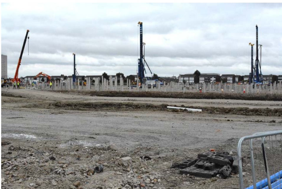
Photo 2-3 Processed WTE bottom ash used as structural base at a construction site in the Netherlands (Photo T Townsend)
