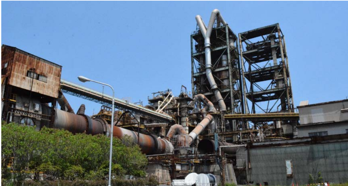
Photo 2-7 Cement kiln in Southern Japan using WTE bottom as a cement kiln feed; this facility washes the ash first to remove salts (Photo: T Townsend)
