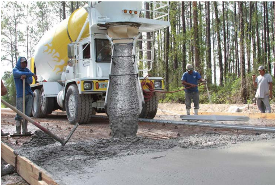
Photo 2-4 Portland cement concrete pavement incorporating processed WTE bottom ash as a partial aggregate replacement in Pasco County (Photo: T Townsend)
