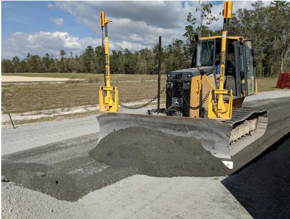
Photo 2-2 Processed WTE bottom ash placed as structural base under a concrete structure in Pasco County Florida (Photo: T Townsend)
