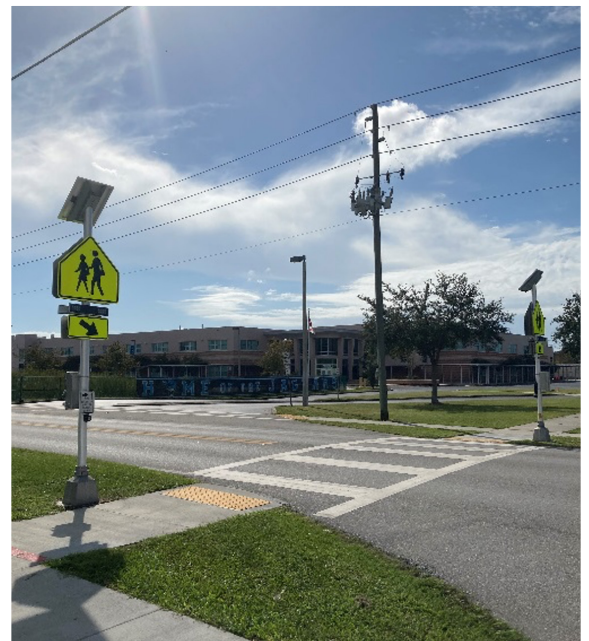
Rectangular Rapid Flash Beacons (RRFBs) installed by Lealman Innovation Academy at 28 th St. N. and 50 th Ave. N.
