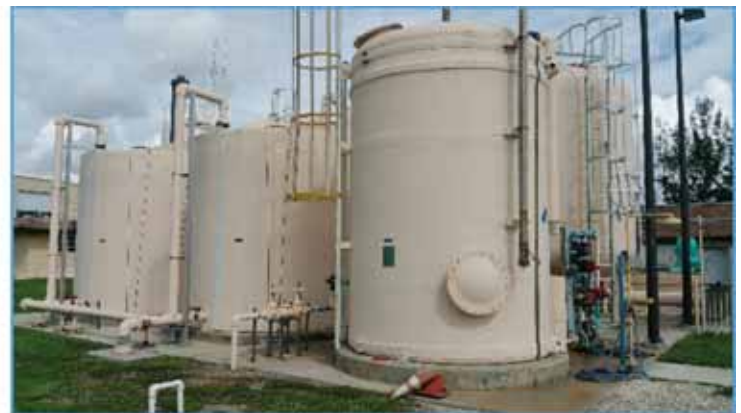
Figure 2. Existing IEX System at the Town of Davie System 3 Water Treatment Plant
