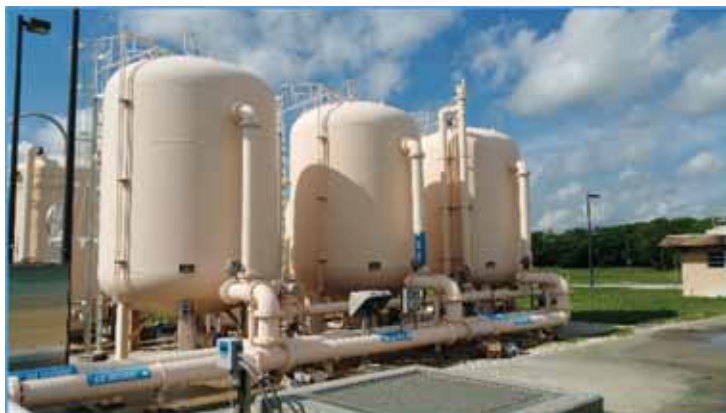
Figure 2. Existing IEX System at the Town of Davie System 3 Water Treatment Plant
