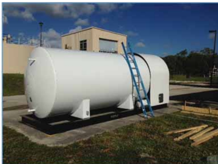
Figure 4. Carbon Dioxide Storage Tank and Dissolution Skid During Construction
