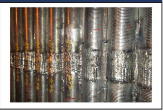
**Project Description:** Replacement of various boiler pressure tube bundles in all three Waste to Energy boiler units.
