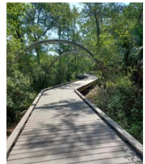
New boardwalk at Brooker Creek Preserve
