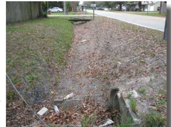
Existing Area Drainage Infrastructure
