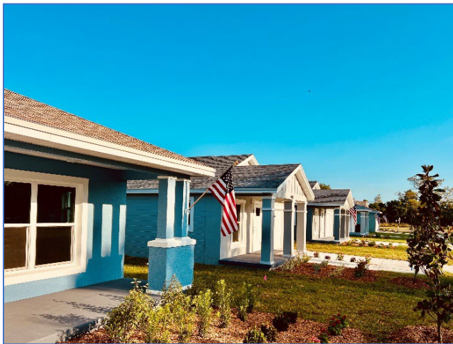
Habitat for Humanity for Pinellas and West Pasco Greenway Habitat homes in the Lealman CRA.
